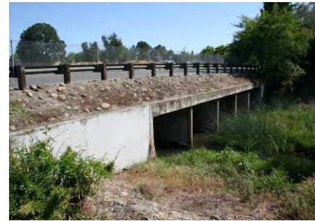
Rocky Ridge Drive multi-cell box culvert at Linda Creek
