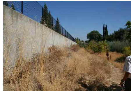
Reinforced concrete flood walls along Linda Creek near Sunrise Avenue
