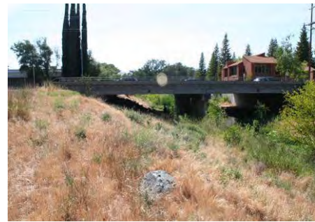
Sunrise Avenue Bridge over Linda Creek
