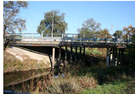
Darling Way Bridge over Dry Creek
