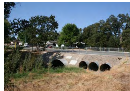
Champion Oaks Drive multi-cell culvert at Linda Creek
