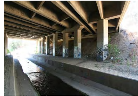
I-80 Bridge over Cirby Creek
