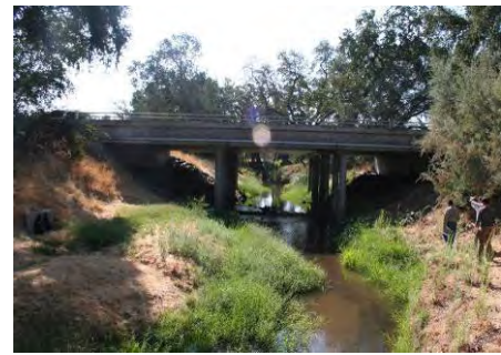
Old Auburn Road Bridge over Linda
