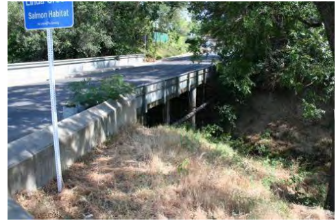
Oak Ridge Drive Bridge over Linda Creek
